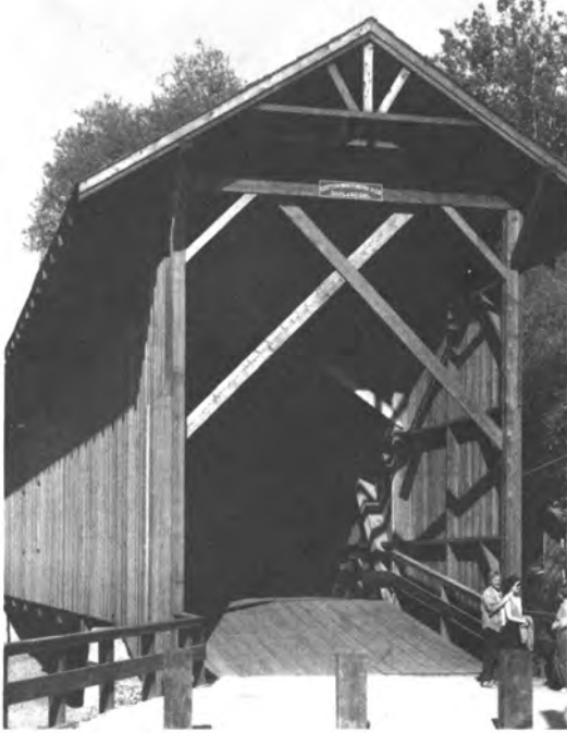
The Felton Covered Bridge in Santa Cruz County -- one of 7 Design Award winners, and a fine example of long-term volunteer effort.
