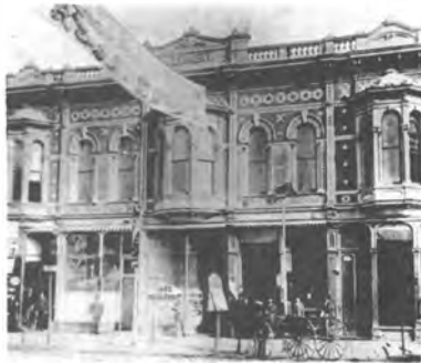
Old Oakland's Leimert Building, as it was and as it is again, thanks to Storek & Storek, Architects.
