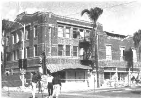
Fillmore's Masonic Temple — red-tagged but repairable — was demolished on February 8 despite a restraining order filed by local citizens attempting to buy some time for a thorough structural study.
