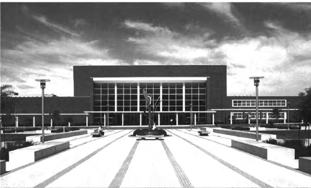
Richmond Memorial Civic Center. Photo: Vern Cheung
