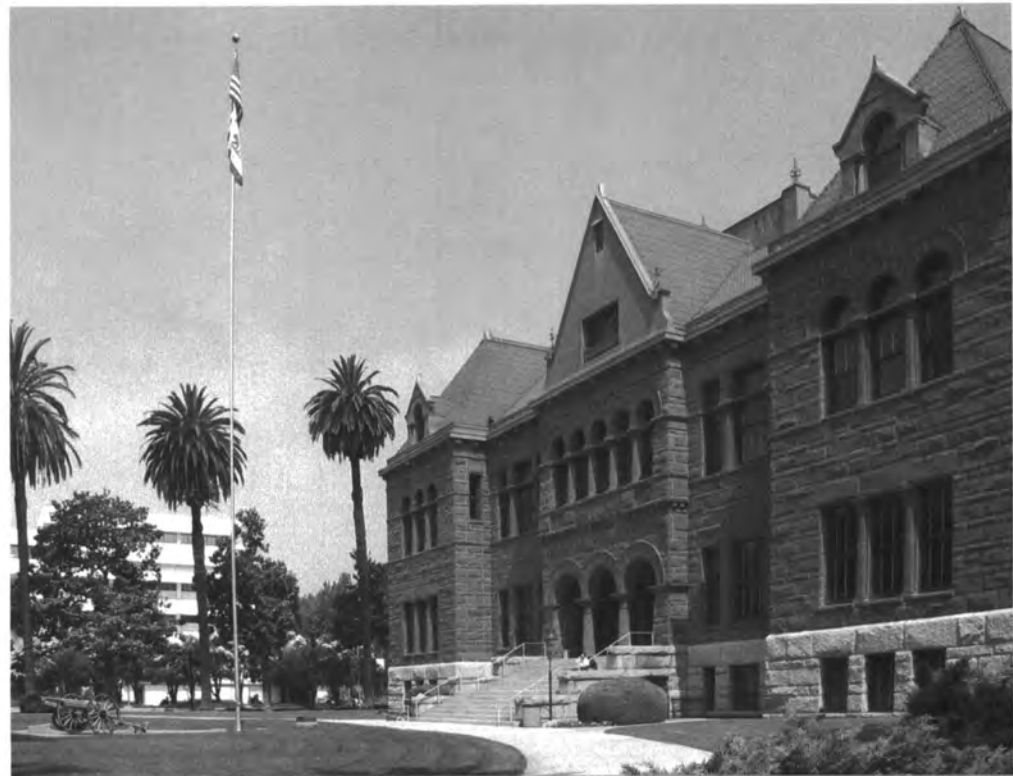
Courthouse. Photo courtesy of Orange County Parks
