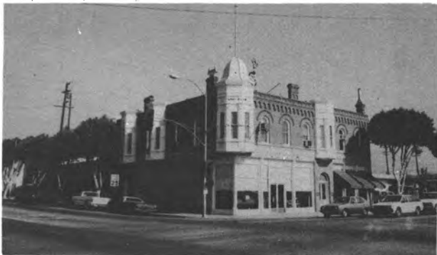
The 1890 building in Santa Paula where Union Oil was born
