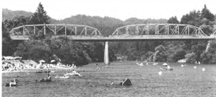
The Guerneville Bridge - listed in the National Register on August 4, 1989
