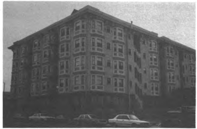
Madison Park Apartments
