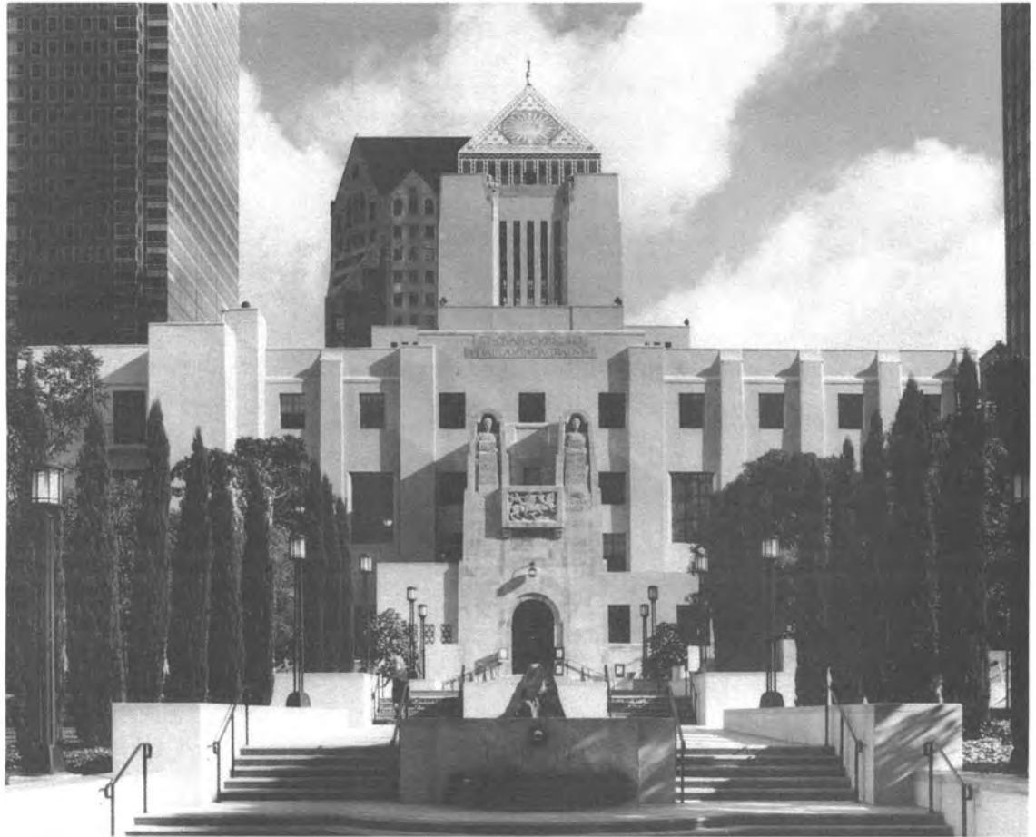
The Los Angeles Central Library (Bertram Goodhue, 1926), site of CPF's 1998 Preservation Design Awards presentation.
