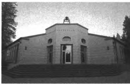
Nevada City Elementary School. Photo: © Justin Nunnink
