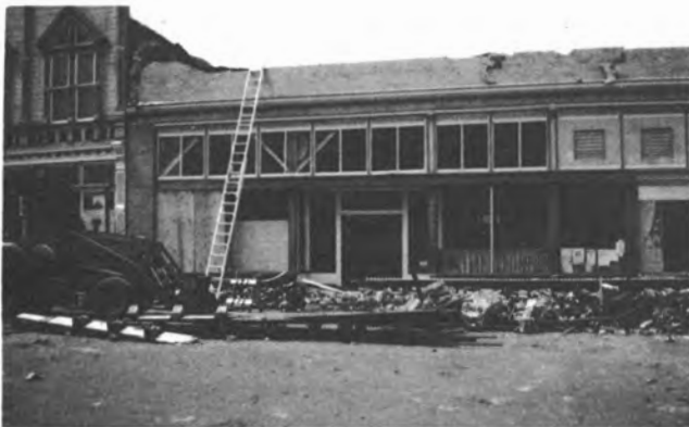
This quake's most-often-photographed building (Fern-dale' Smith Grocery) was ultimately demolished despite efforts to convince owners that it was an "easy fix." (photo credit: David Cocke)
