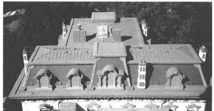
Stanford Mansion Roof upon completion of Phase I
