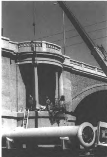
North Broadway Viaduct/Bridge in Los Angeles, during restoration
