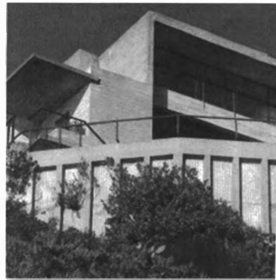
Haliburton House, Photo credit: Alan Hess.
