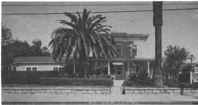
Upham Hotel , 1404 De La Vina Street, Santa Barbara, CA 93101, 805/962-0058; 800/727-0876
