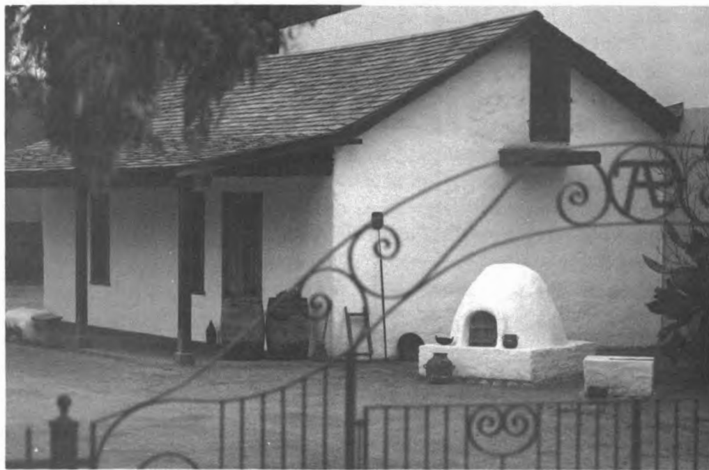
The Peralta Adobe, San Jose
