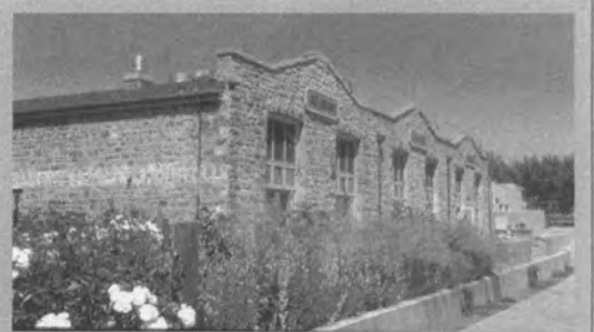
c.1895 Williams building on Main Street in Napa, saved by recent seismic retrofitting
