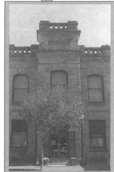
The City of Napa is planning additional seismic retrofitting for the Goodman Library, c. 1901, that it owns.
