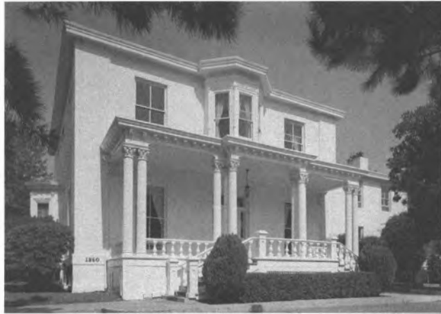
The Commanding Officer's Quarters (1860) is one of six mid-19th century structures vacant and suffering from deferred maintenance.
