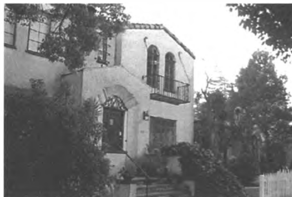
Hacienda Gardens, saved from demolition by the San Carlos Heritage Association.
