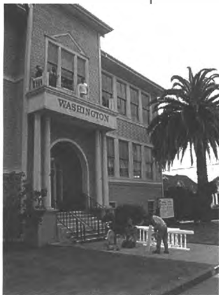
Students of the College of the Redwoods' HPRT Program reconstructing the balustrade of the Senior Resource Center in Eureka.
