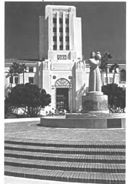
County of San Diego Administration Building, awarded an "Orchid" for its sensitive restoration.
