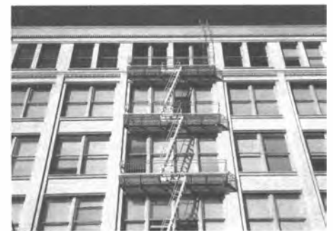
Merritt Building San Francisco, San Francisco County Owner: William Lightner, Millennium Play, LLC Costs: $6,550,000
