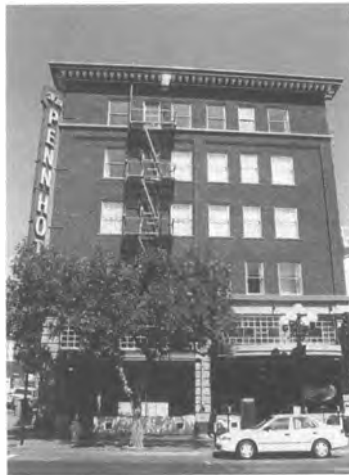
Oxford Hotel, aka William Penn Hotel San Diego, San Diego County Owner: William Penn Hotel, LLC Costs: $4,611,054
