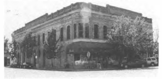
Devilbiss Hotel/ Buckhorn Restaurant Building Woodland, Yolo County Owner: John Pickerel, Houkan Dissbee Partnership Costs: $458,708
