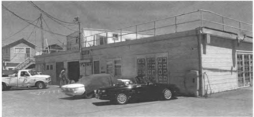
WWII ship launch and buildings now serve as shop space for local maritime trade
