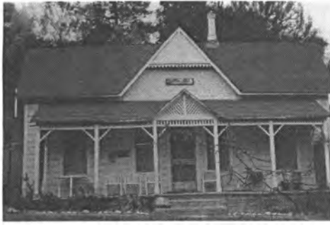
Buena Vista Cottage, demolished in November 2003
