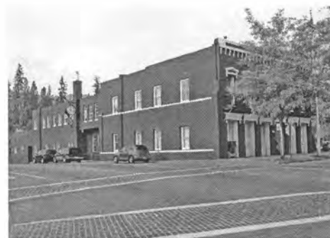
Trinity County Courthouse (1856-57), Weaverville; Photo: Mike Weininger, The Trinity Journal
