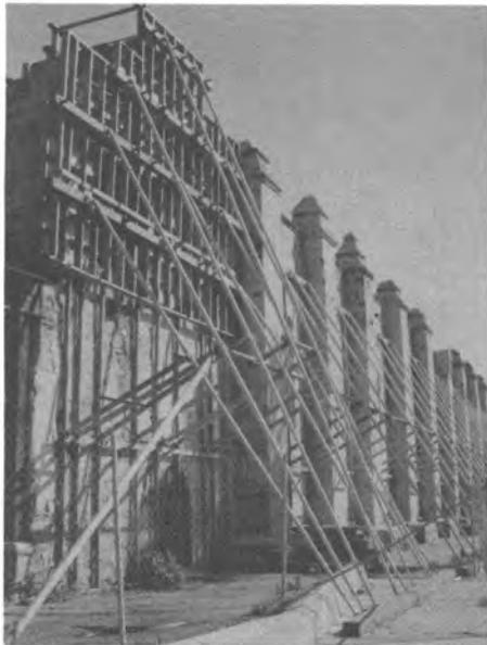
The 1987 Whittier Quake caused great damage and closing of the Mission, one of California's oldest extant structures. The Getty grant will finance emergency repairs to prevent the collapse of the mission's structure as well as a detailed structural analysis for conservation sympathetic to its architectural history.
