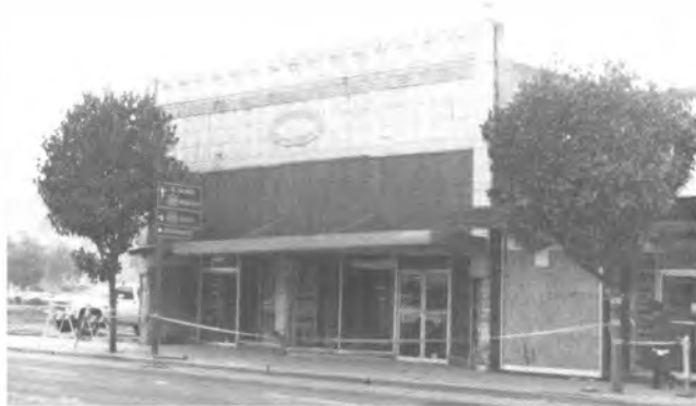
A building in Watsonville "red-tagged for months and nearly demolished for no apparent reason.
