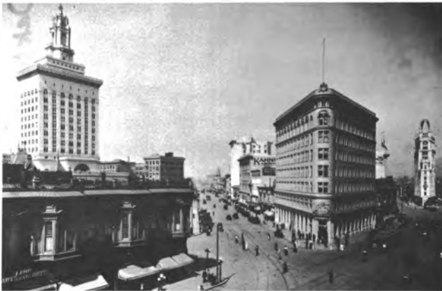
City Hall (left), the Broadway Building (center) and CPF's Cathedral Building (right): historic photo (circa 1914) courtesy of the Oakland Museum
