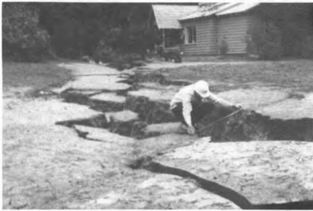
Photo: Richard Eisner, Bay Area Regional Earthquake Preparedness Project
