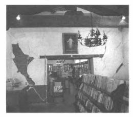
Concrete bond beams were anchored to roof rafters in the Major Domo's House. The plaster in the House and the Museum Building was repaired or replaced and these walls were also injected with modified mud. The stabilization and repair retained historic fabric and ensures the continued presence of one of the most important reminders of a vanished period in California history.
