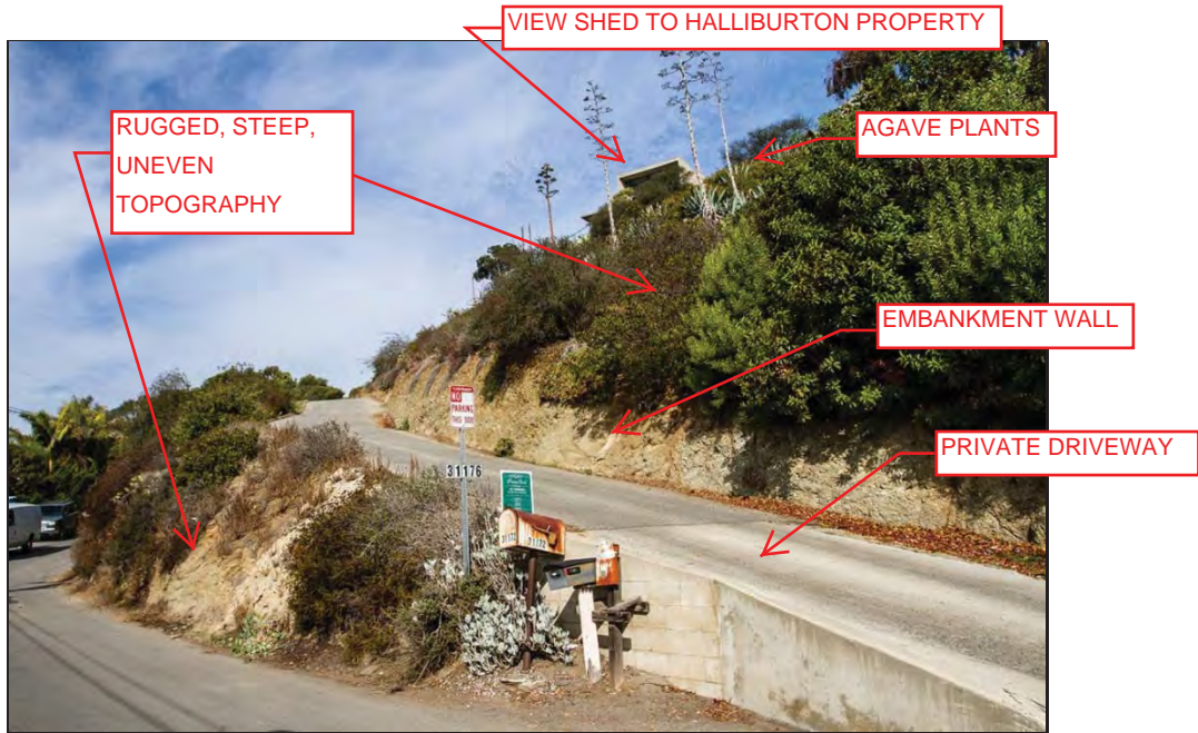
Circulation Features and Topographic Characteristics, 31204 Ceanothus Drive
