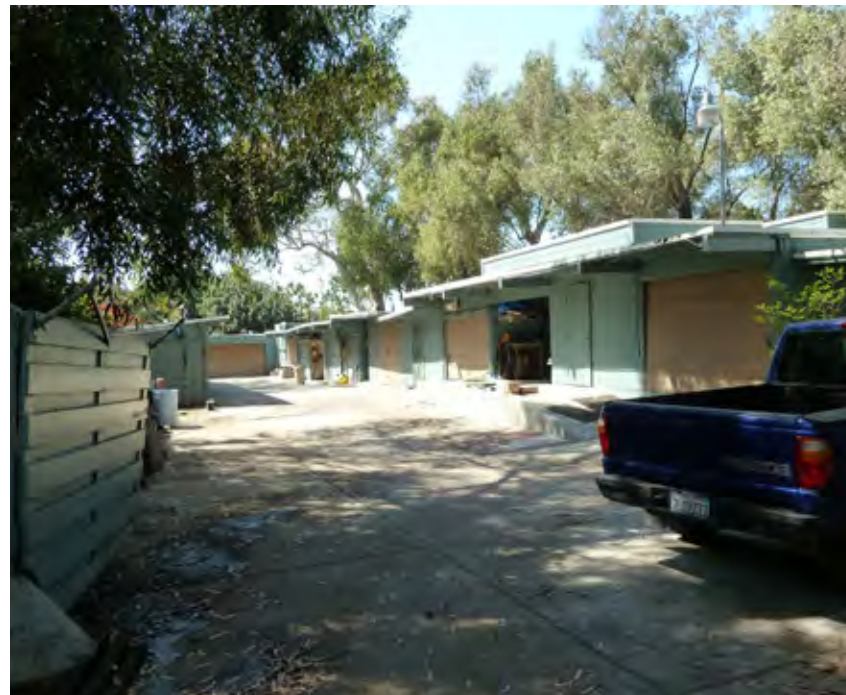
Maintenance Shed, Building 97, 2013. (Photo by Holly Kane)
