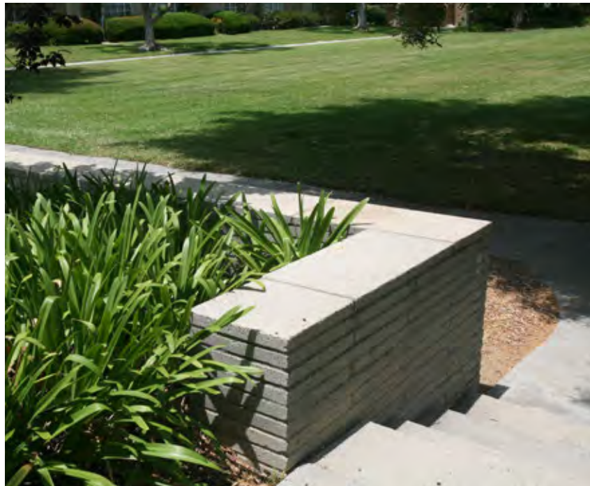
Rear view of wall in Court 4/5 showing that the wall is a design element heightening horizontal motif in the landscape rather than a truly functional retaining wall, 2013. (Photo by Holly Kane)
