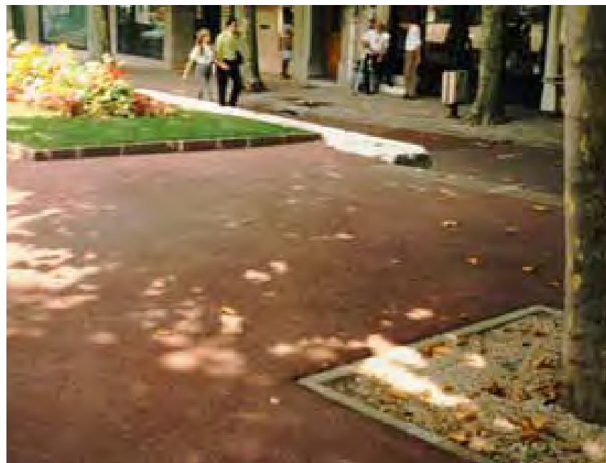
Example of colored asphaltic concrete paving
