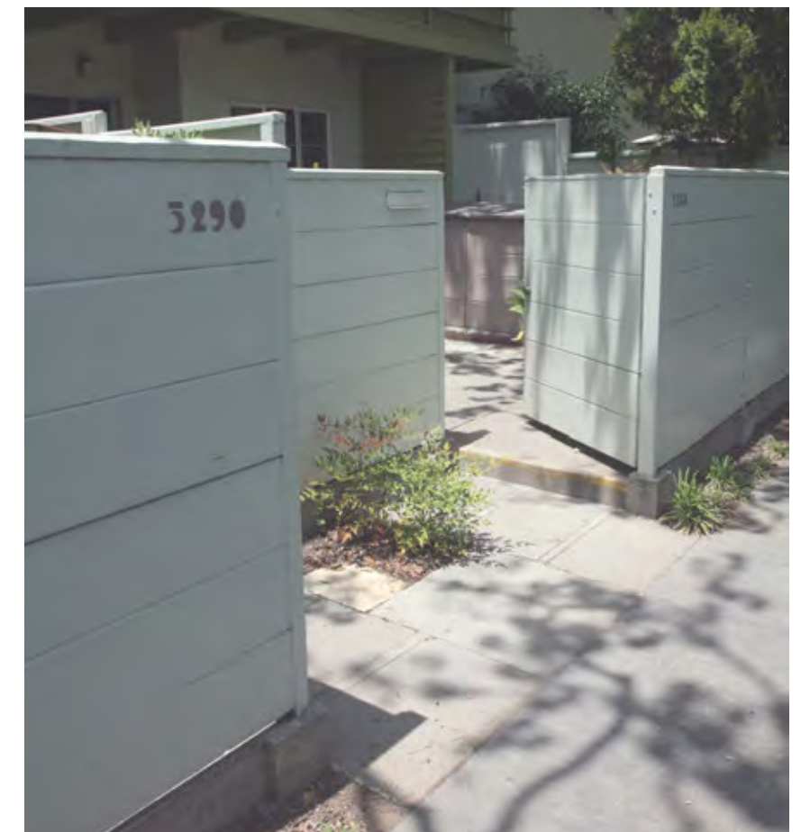
Pavers in patio and patio entrance in Garage Court 4, 2013. (Photo by Holly Kane)
