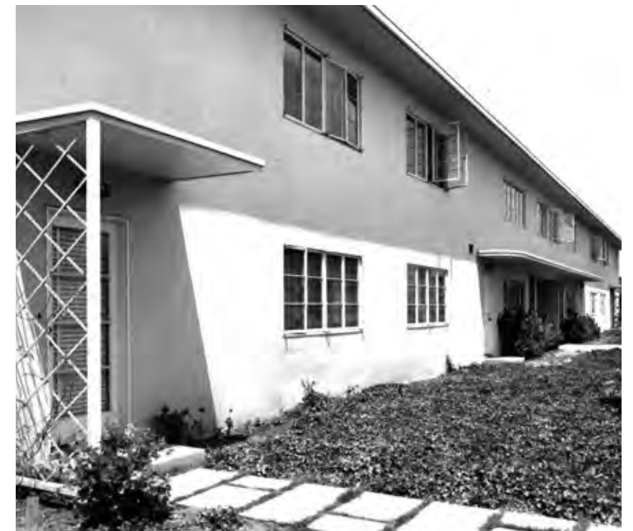
Note the trellis next to the formal entry, designed to be covered by a vine, original concrete paving stones leading to entry, and groundcover next to building, 1942. (Photo by Margaret Lowe, Robert Evans Alexander papers, #3087. Division of Rare and Manuscript Collections, Cornell University Library)
