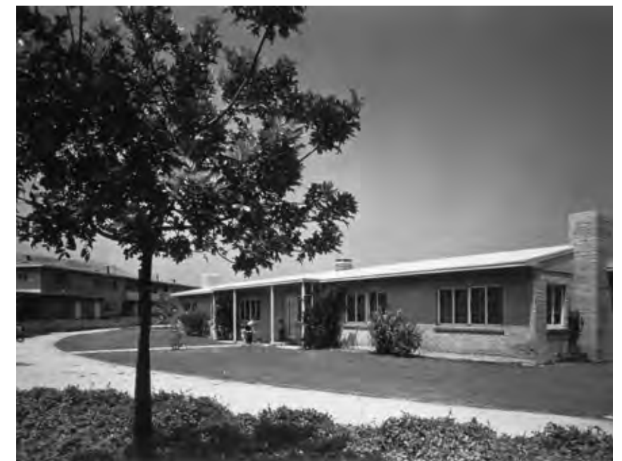
Building 46, Court 9, a bungalow, circa 1944.
