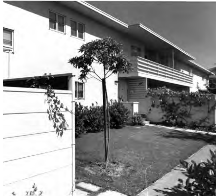
Garage Court side of building showing enclosed patio and open space, early 1940s. (Photo by Margaret Lowe, Robert Evans Alexander papers, #3087. Division of Rare and Manuscript Collections, Cornell University Library)
