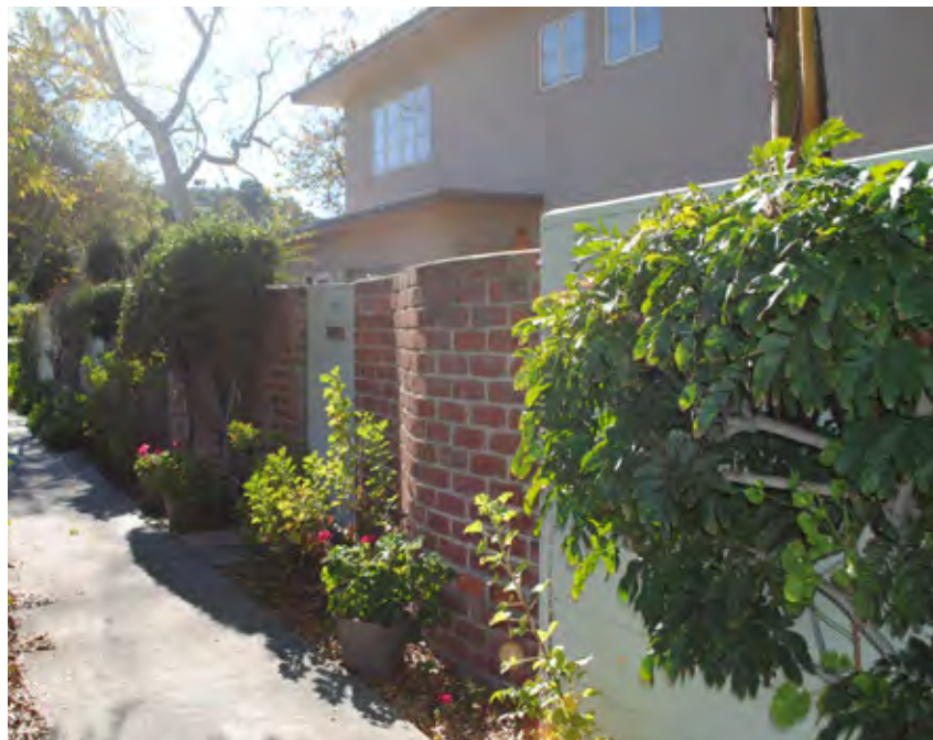
Preserve wood-framed and brick walls, 2013. (Photo by Mundus Bishop)
