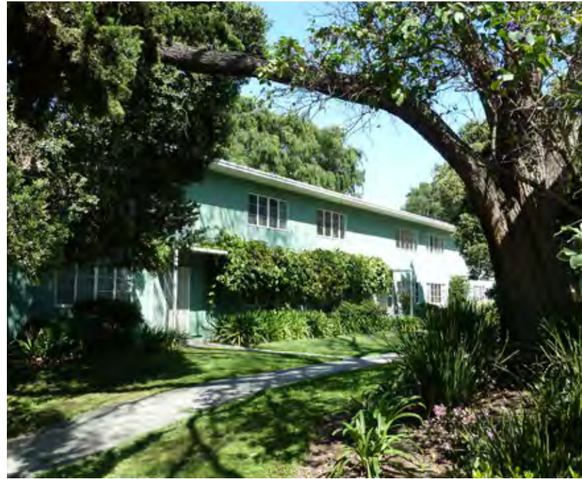
Building 90, a Type 4 building, showing vine growing on horizontal trellis, 2013. (Photo by Holly Kane)
