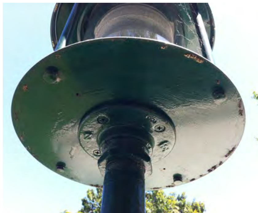
Underside of new lamp posts shows distinguishing features: a number 2 and CSI enclosed in a diamond shaped box, 2013. (Photo by Holly Kane)
