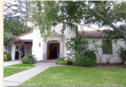
3. Beverly Hills Women's Club, 1925 Architects: Gable & Wyant
