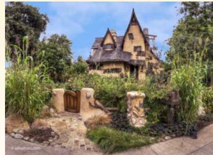
8. The Witch's House, 1920 Architect: Harry Oliver
