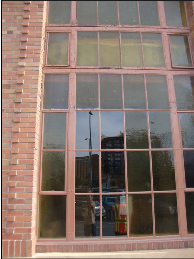
Glazing putty repair
