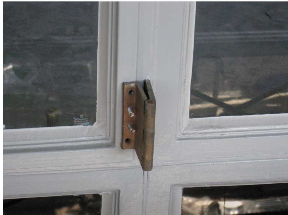
Wet sealant repair
