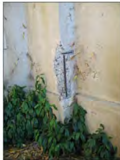
The corroding metal exposed by this large spall was sufficiently covered by concrete. The concrete is dominated by large aggregate, which inhibits cohesion of the matrix.
