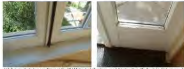
At left, typical window conditions at the Old Union include minor wood deterioration. On the right, historic wood door components near grade exhibit moderate wood decay, as far as this side light at the east elevation. (Source: ARG, 2012).
