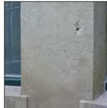
After the patch dried, liquid stains were applied to complete the visual integration of the repair material with the original plaster.
