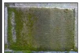
Area II, shortly after application of biocides. (ARG, 2012)
