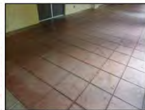
Map cracking throughout the pavement is the result of faulty installation. (ARG, 2012)
