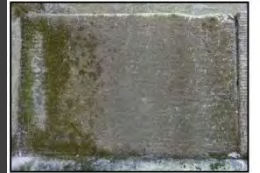
Area II, before application of biocides. (ARG, 2012)
