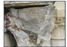
Brick fragments are visible in the spalled patch at a south tower column capital. (ARG/CS, 2011)
