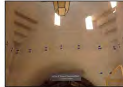
Blue tape was placed alongside test areas at a large horizontal crack at the south tower during a recent plaster assessment. (ARG/CS, 2011)
