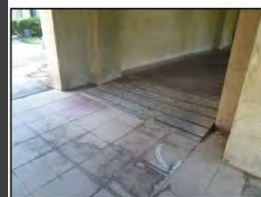
The plywood exterior ramp at the west arcade is in poor condition, but is in compliance. (ARG, 2012)
