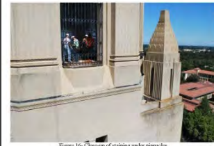
Figure 16- Close-up of staining under pinacles.
