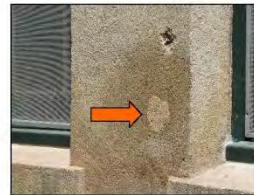
A custom color patching plaster was applied to test areas and scraped level with the surrounding plaster, then left to cure.
