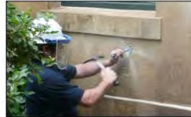
Test patch areas were squared off with a grinder and chiselled to receive the patching material.
