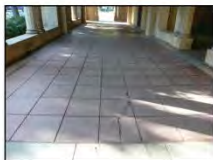
Pavement is cracked and buckled at the south elevation. (ARG, 2012)
