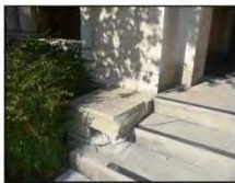
Concrete steps at the south end of the east elevation are cracked and spalled. (ARG, 2012)
