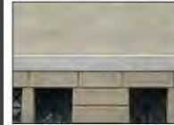
Exterior concrete walls are covered with colored and scored cement plaster, while the rusticated basement wall finish was cast in place and tooled. (ARIG, 2012)
