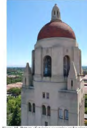
Figure 15- Pattern of staining occurring under pinacles.
