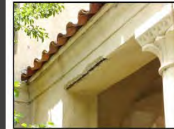
Corroding reinforcing metal is exposed at this concrete spall adjacent to the south tower. (ARG, 2012)
