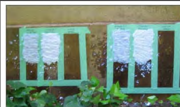
Cleaning test panels were created to assess leaving light red staining left and heavier red staining right. In each panel, a cleaning practice of ammonium citrate is on the left, a water practice is in the center, and repeated water spraying took place on the right.
