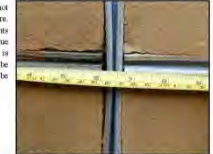
Deteriorated plaster panels cannot be easily repaired, and will eventually need to be replaced. (ARIG, 2012)
