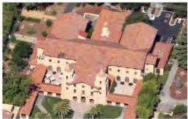
This aerial view of the Old Union clarifies the complicated footprint of the building. The east wing projects out from the center core, creating two side courtyards, while three additional wings extend out at the rear facade. (Source: Google Maps, 2012)
