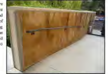
Stains and biologic growth should be cleaned before carrying out preventive lapping or coating of walls. (ARIG, 2012)
