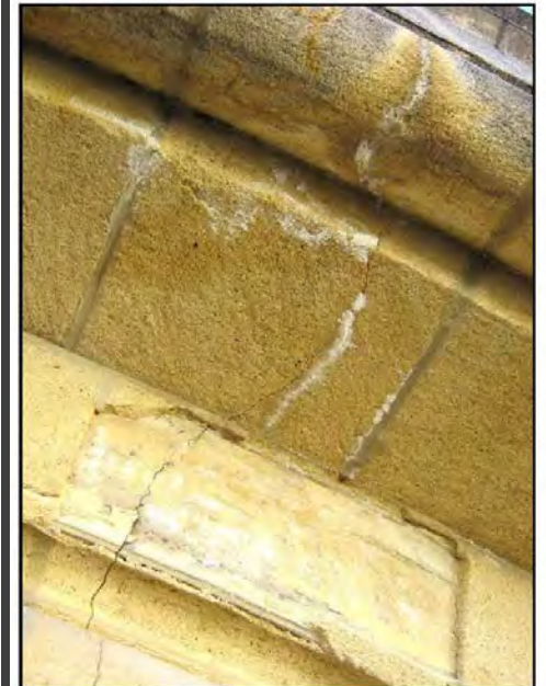
Plaster de-bonding is associated with cracking and efflorescence at the south tower arches. (ARG/CS, 2011)
