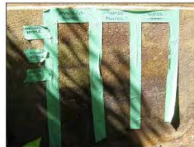
All of the tested methods removed some staining, but the ammonium citrate was the most effective material, removing significant staining using relatively gentle tools.
