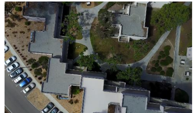
Dorm inspection at UC San Diego
