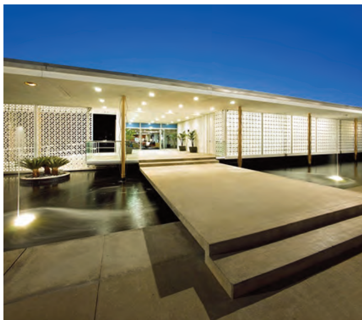
The Stuart Building. BRE professional photograph.
