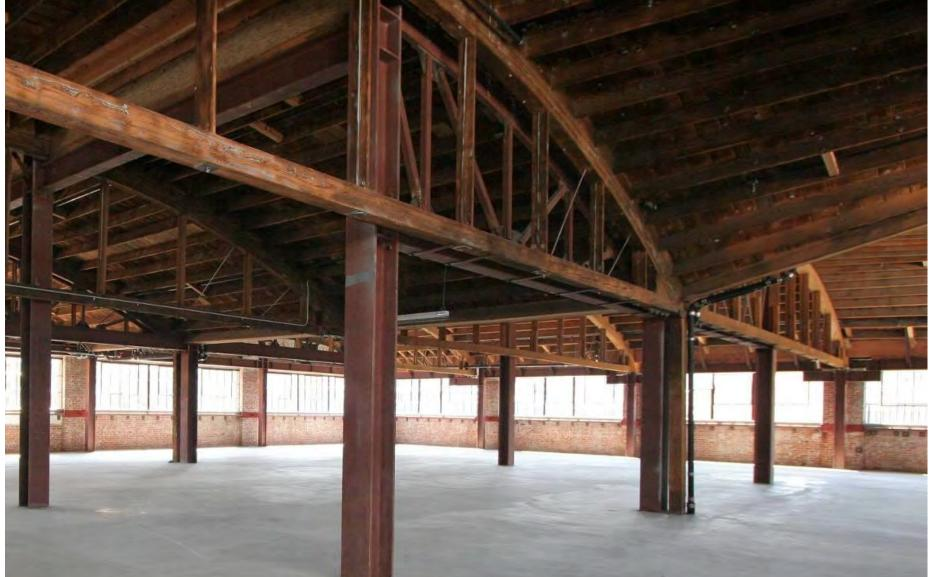
Originally built of unreinforced load-bearing masonry, a steel skeleton was carefully inserted to give the building additional strength and seismic stability. The historic timber members remain.
