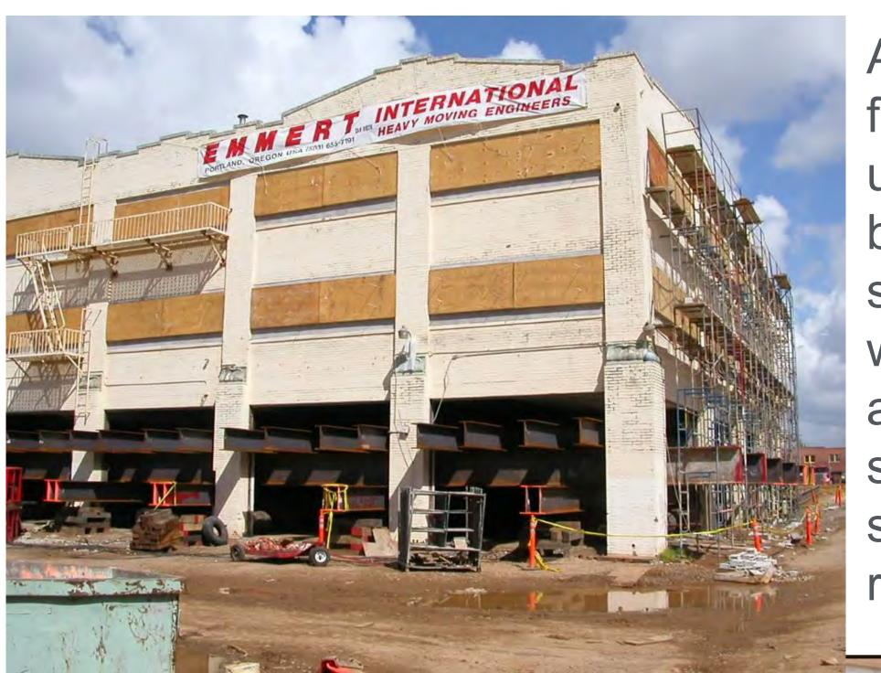
A steel supporting frame on dollies was used to carry the building to its new site. The first floor was disassembled and the bricks and storefronts were stored for later rehabilitation, 2004.
